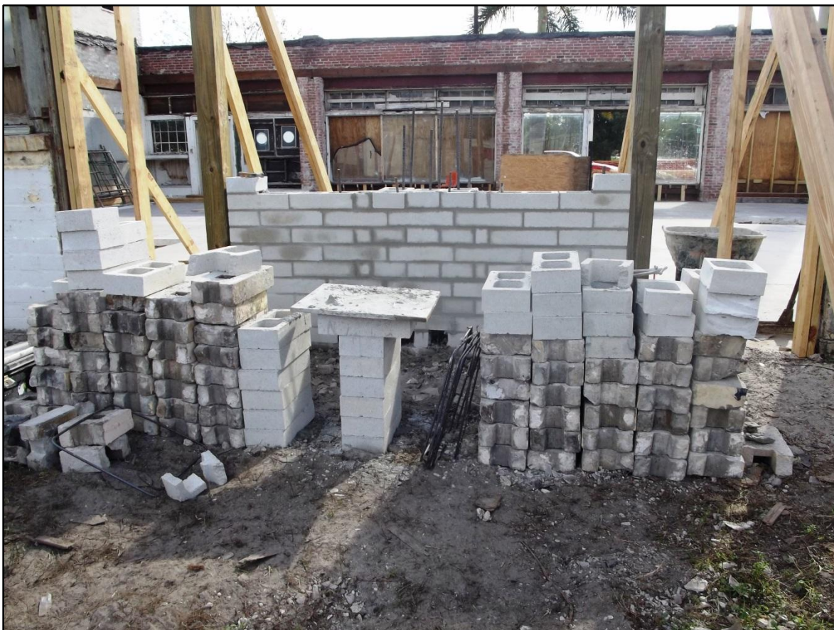
View from outside: reconstruction of the damaged portion of the rear wall
