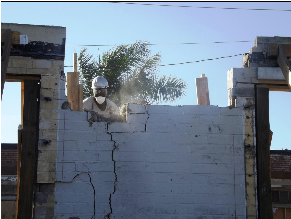
View from inside: demolition of damaged portion of rear wall
