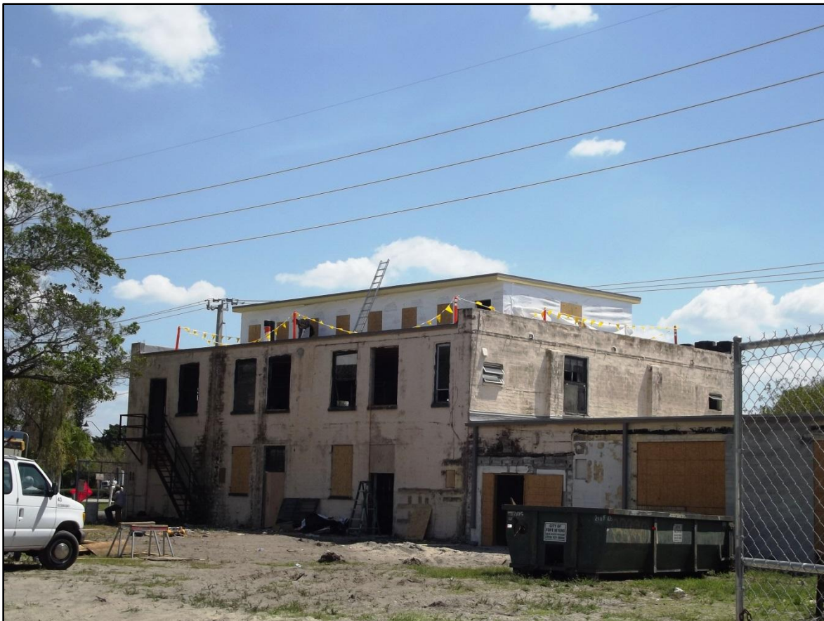
View from rear: roof reconstruction
