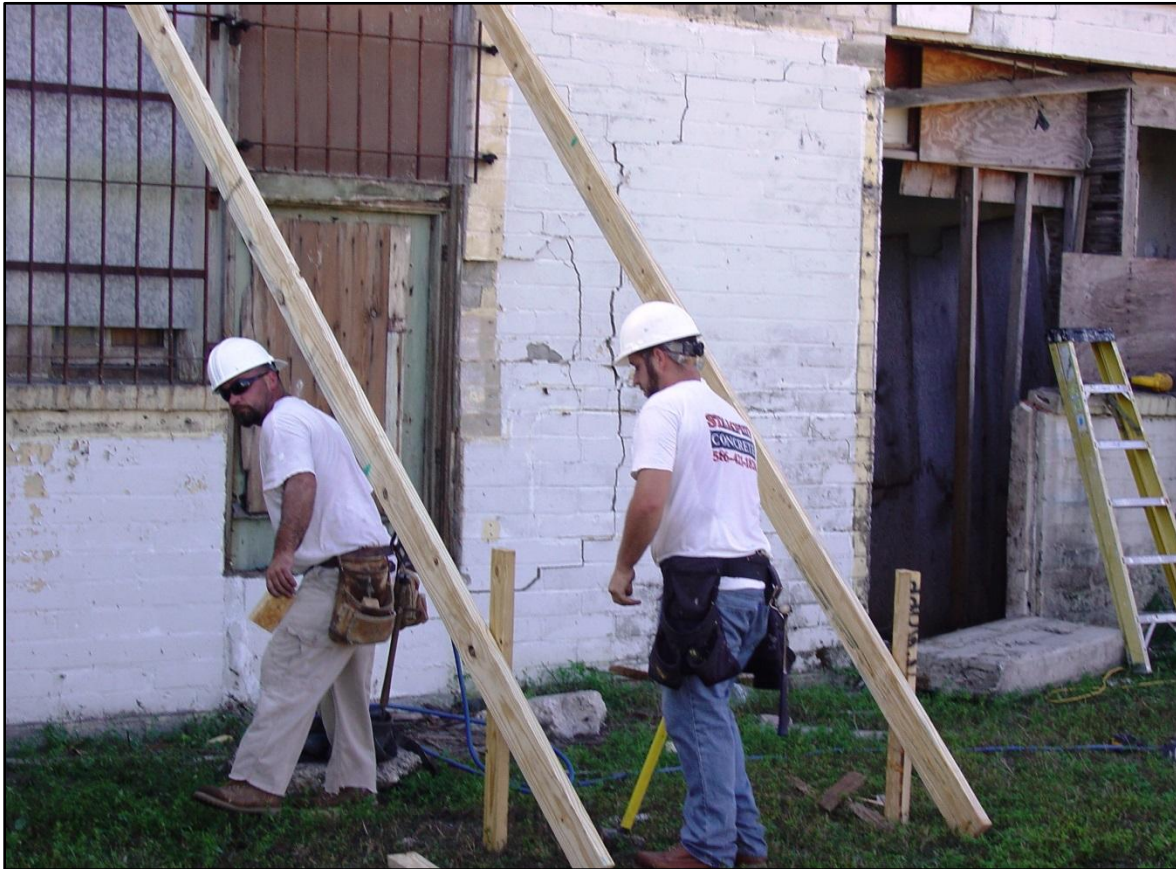
View from outside: rear wall shored up in preparation for the damaged section to be replaced
