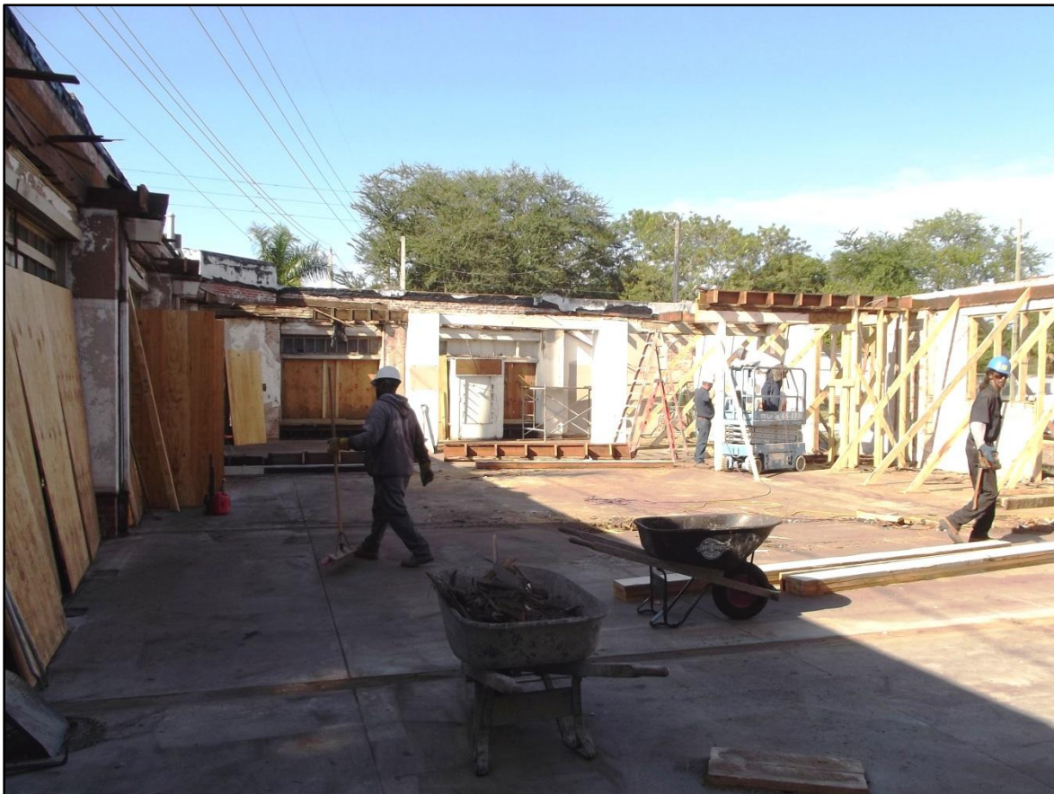
View from inside the 1-Story building: the entire roof has been removed
