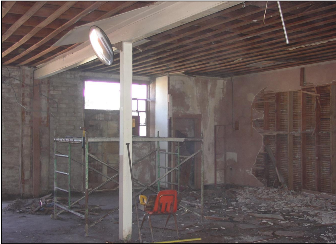
View from inside the 1- Story building : interior demolition
