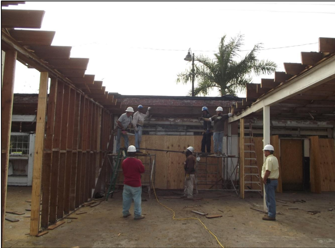
View from inside the 1-Story building: roof section removed
