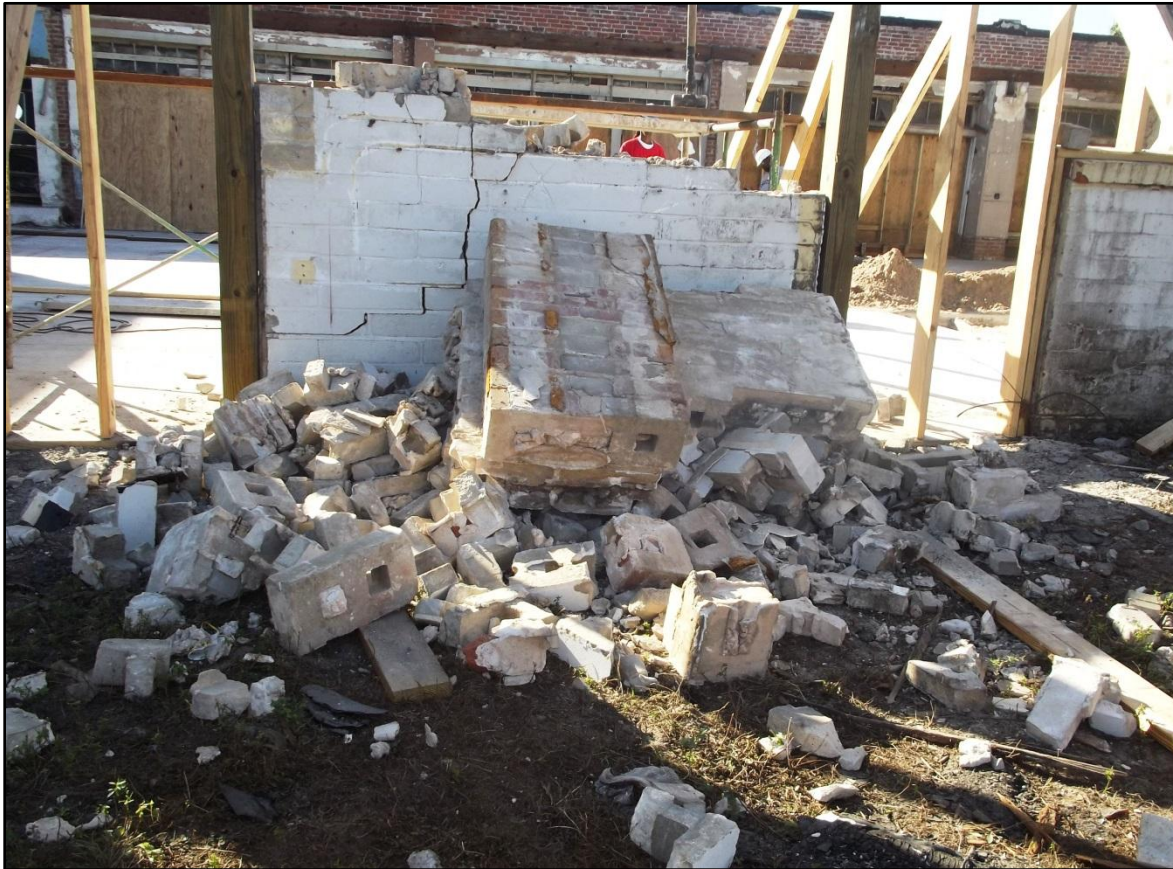
View from outside: demolition of damaged portion of the rear wall
